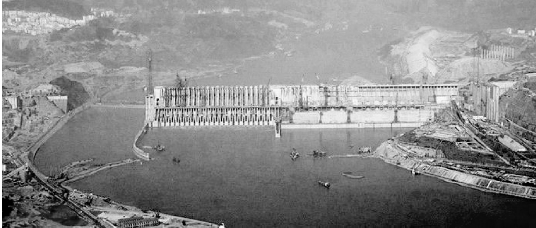
Fig. 4. Downstream view of the Three-Gorges Project under construction.
