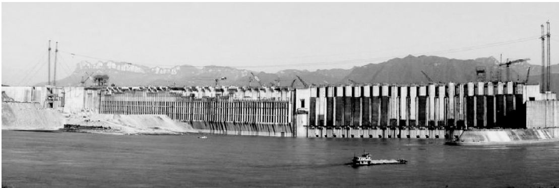
Fig. 3. Upstream view of the Three-Gorges Project under construction.
